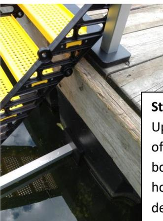
**Step 3** - Attach the Upper Mounting Plate with Warning Label to the tapped end of each Upper Mounting Leg using the two (2) 5/16-18NC button head cap screws provided.
